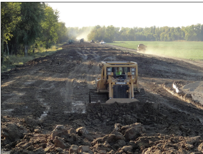
A Vicksburg-based crew repairs a 300-foot-long washout near the lower crevasse Sunday.
