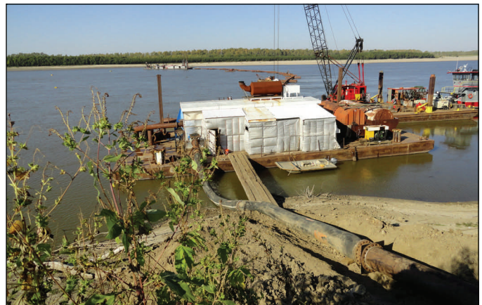
The dredge (background) pumps sand to a booster pump (on barge, center), to the shore pipeline via a section of flexible pipe (foreground), and then to the scour hole at the center crevasse.
