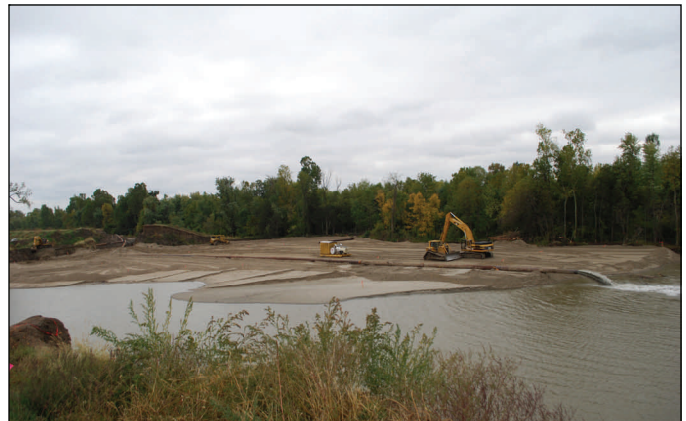
The dredge contractor pumps sand into the scour hole at the center crevasse Wednesday.
